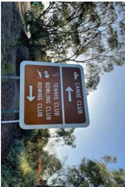
Chaffey/Cureton Ave - Incorrectly signed and positioned community facility sign (should be a blue sign)
