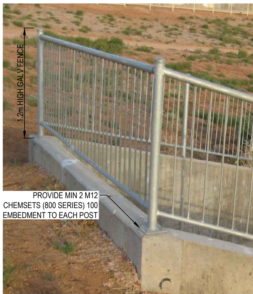
TYPICAL HEADWALL FENCE
