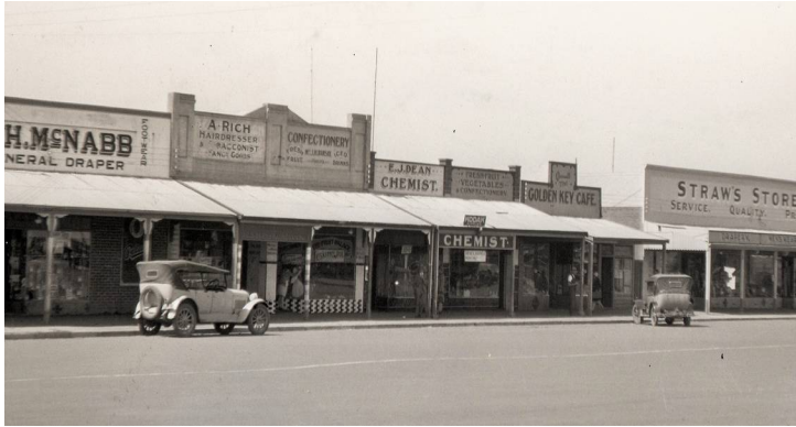
Indi Avenue, North side, circa 1925 Shop verandah roofs are steeply sloping with timber posts. Variety of large signs on parapets
