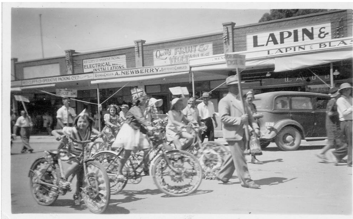
Ilex Street, East side circa 1955 Verandahs cantilevered (no posts) Variety of large signs on parapets.
