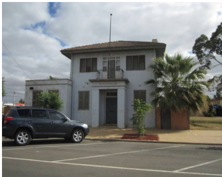
22 Ilex St. (Former Bank of NSW)
