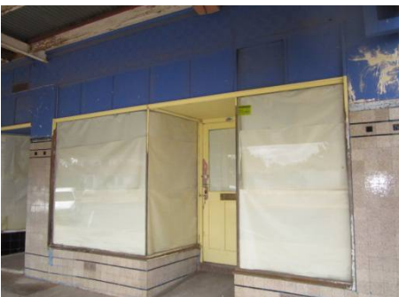
39 – 41 Ilex St. Remove paint off glass above door heads shopfront.
