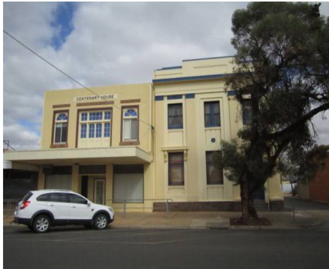
48 & 50 (Former Commonwealth Bank ) Indi St. Examples of preferred colours for major items (Indi Ave.) Cream walls with red or green trim,
