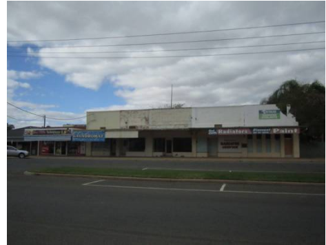
67 – 69 Ilex St. Paint parapet, Portland Stone with boarders darker tone.
