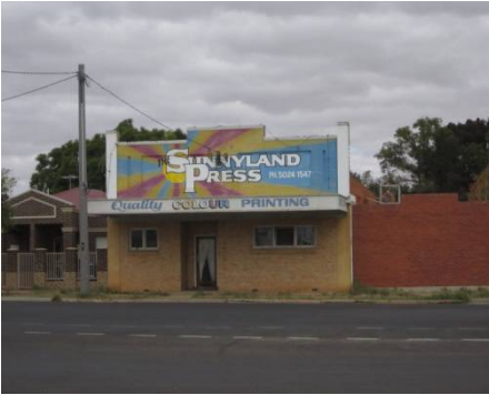
18 Jamieson St. Reduce impact of sign, Paint border, Portland Stone
