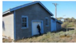
Relift Pumping Station, Walpeup
