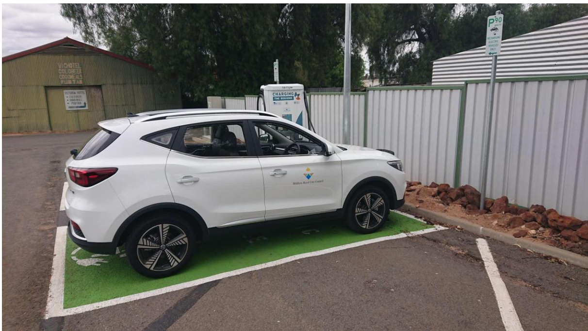
Figure 1: Public EV Fast Charger at Ouyen Community Park
