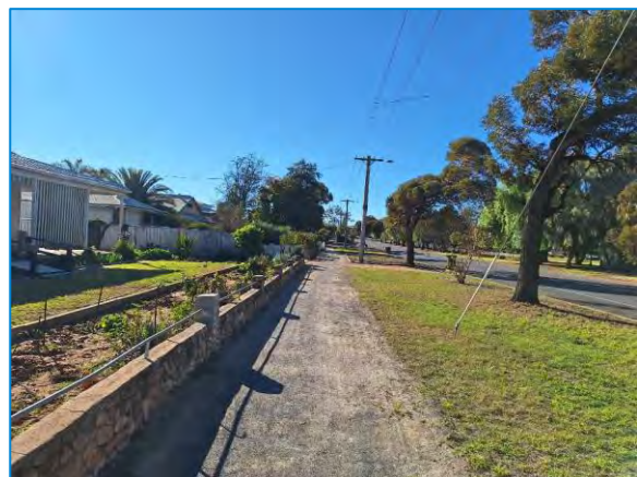
Figure 8: Gypsum Footpath - Oke Street
