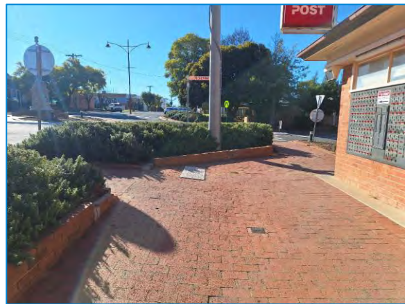
Figure 6: Paved Footpath - Oke Street
