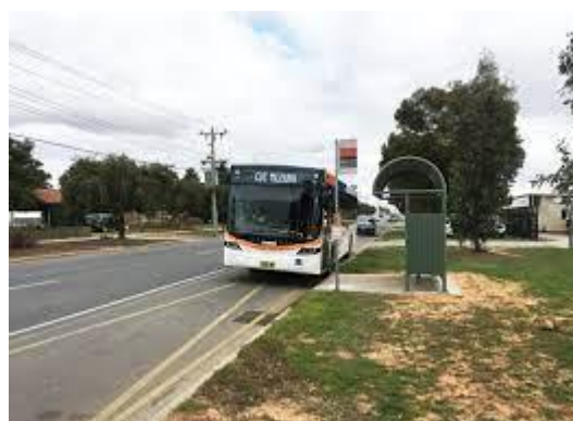
Figure 1 – Example bus stop in Mildura
