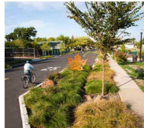
Example of a mid-block pinch-point
