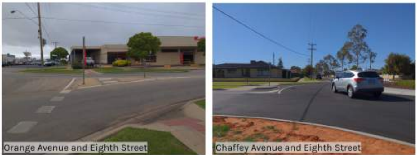
Figure 22 Untreated Roundabout Crossings
