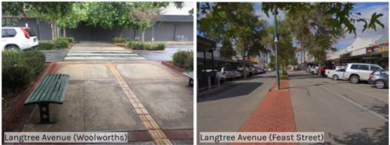
Figure 19 Mid-block raised zebra crossing
