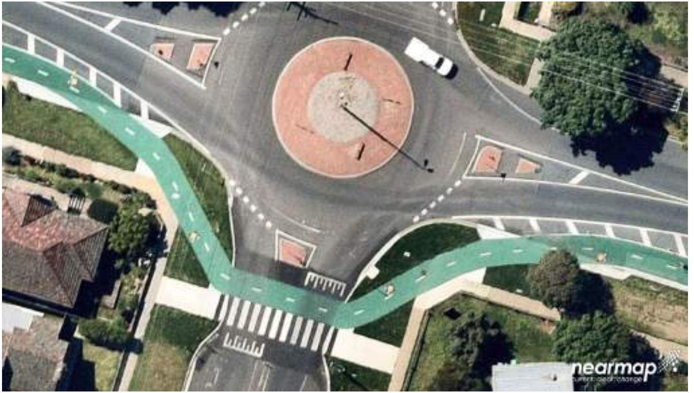
Figure 38 Protected roundabout in Bendigo
