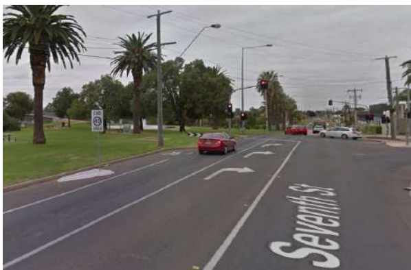
Figure 29 Road Furniture in the bike lane
