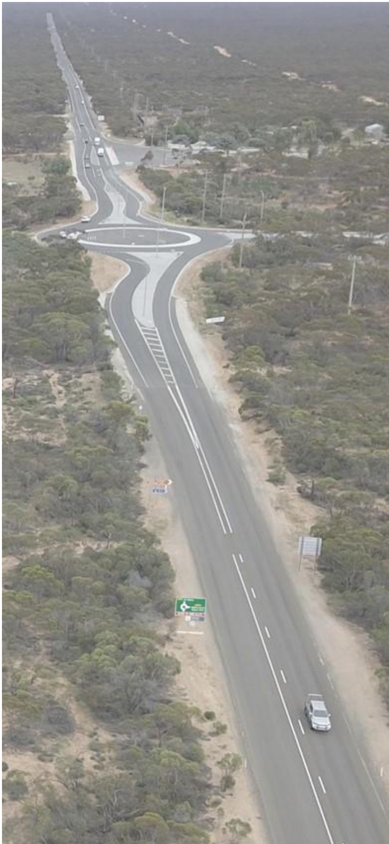
Figure 6-6 New round-about at intersection of Calder Highway and Hattah-Robinvale Road (looking north along Calder Highway) 18
