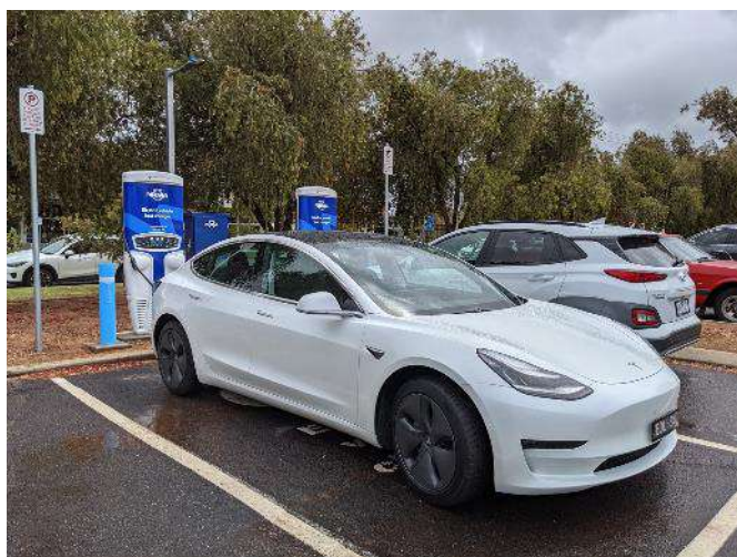
Figure 49 Council has installed fast chargers in the CBD
