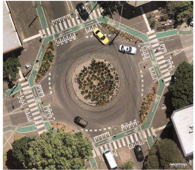
Figure 32 Raised zebra roundabout, South Melbourne
