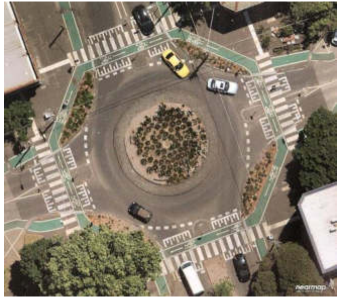
Figure 32 Raised zebra roundabout, South Melbourne
