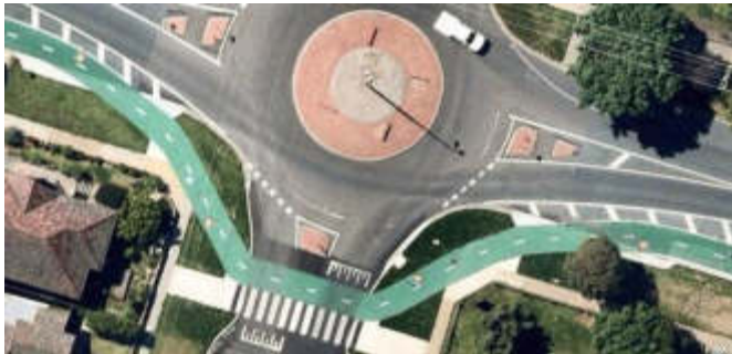
Figure 27 Protected roundabout, Bendigo
