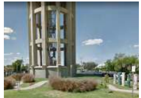
A8 Mildura Water Tower
