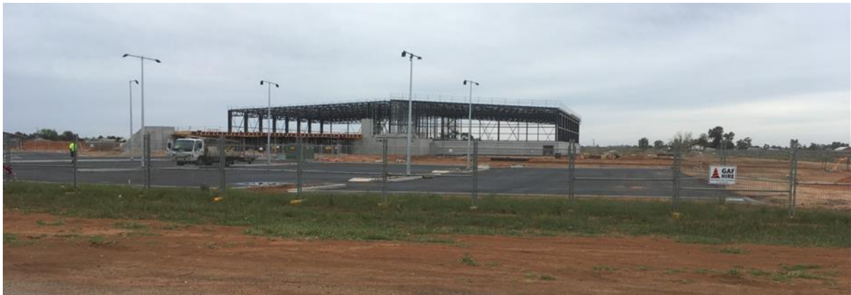
Figure 6 MSRPSP indoor stadium and carpark areas under construction
