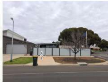
Figure 5 Site affected by the DDO11
