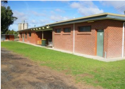
Social / multi-purpose room and public toilets (right end of building)
