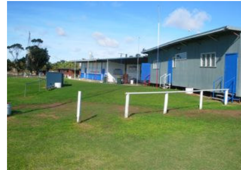
Football / cricket change rooms (right end of building) and kiosk / shelter.
