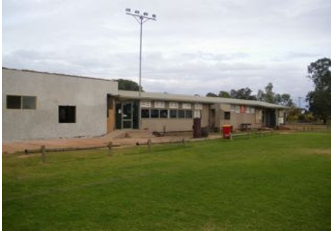
Old and new sections of pavilion
