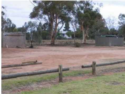
Old toilet blocks - to be demolished on completion of new public toilet facilities
