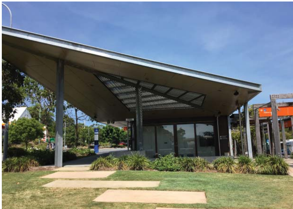
Image 33 Noosa Junction Bus Station (QLD) is a transport hub, meeting place and landmark
