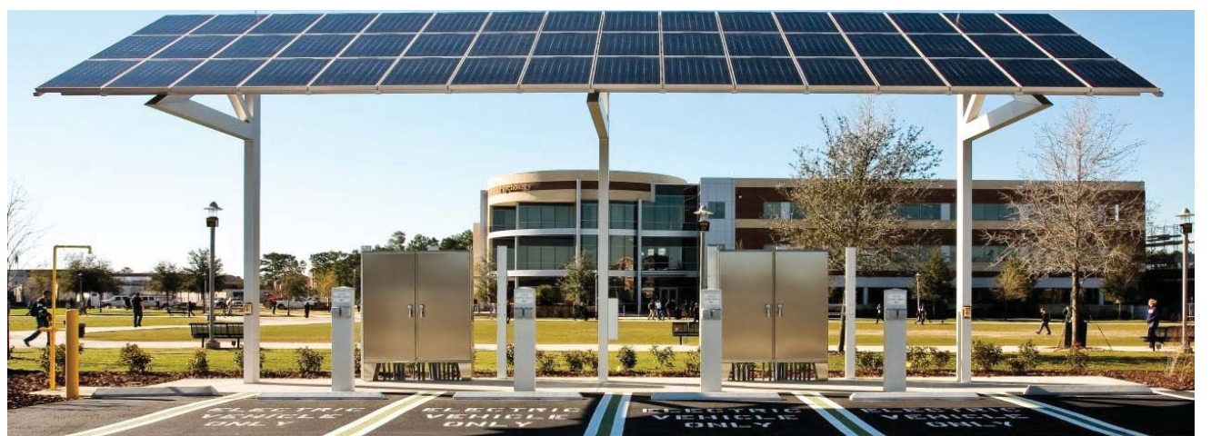
Image 54 Solar powered electrical charge points (University of Central Florida, USA)
