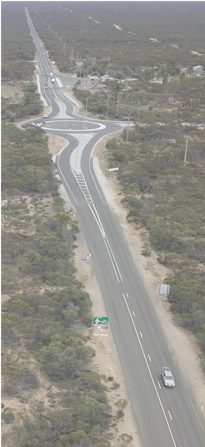
Figure 6-6 New round-about at intersection of Calder Highway and Hattah-Robinvale Road (looking north along Calder Highway) 18
