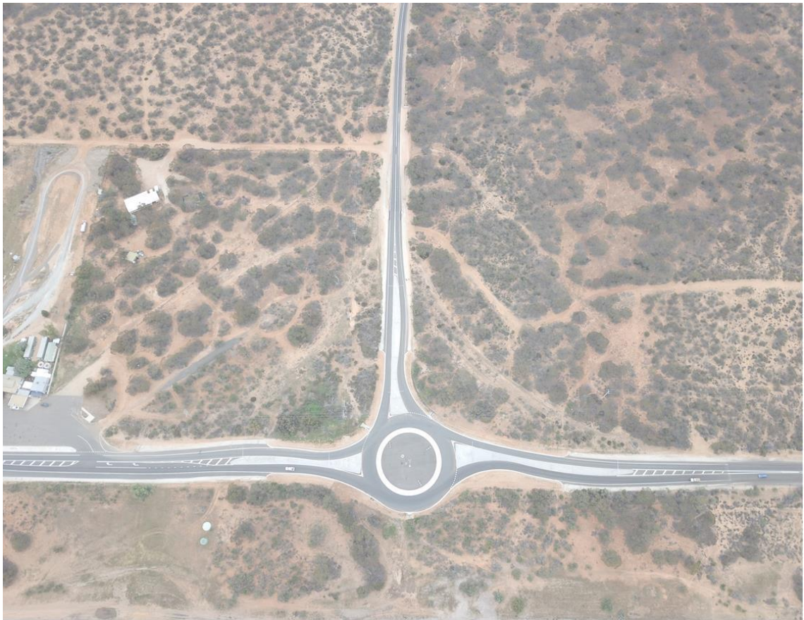
Figure 6-7 New round-about at intersection of Calder Highway and Hattah-Robinvale Road (looking east along Hattah-Robinvale Road) 19
