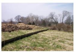
Figure 7 - Silt Fence (US EPA 2008)
