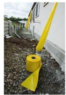
Figure 2 - Temporary Downpipes
