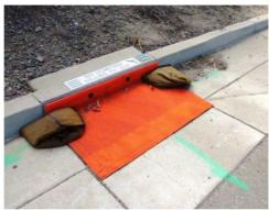
Figure 3 - Sediment Trap
