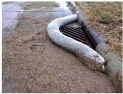
Figure 5 - Sediment Trap
